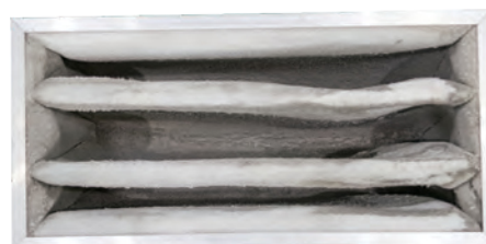
The filter that needs to be replaced
